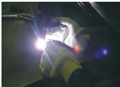
Use of advanced technique on Tungsten Inert Gas Welding.
